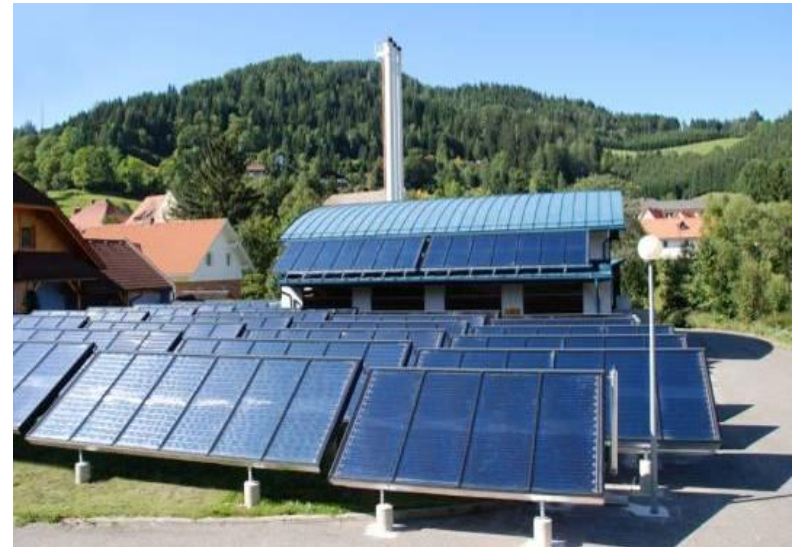
Post mounted system, Oberzeiring, Austria [SOLID]
